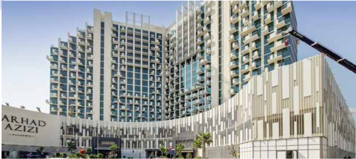
AZIZI RESIDENTIAL BUILDING G+ 2P+17F DUBAI
